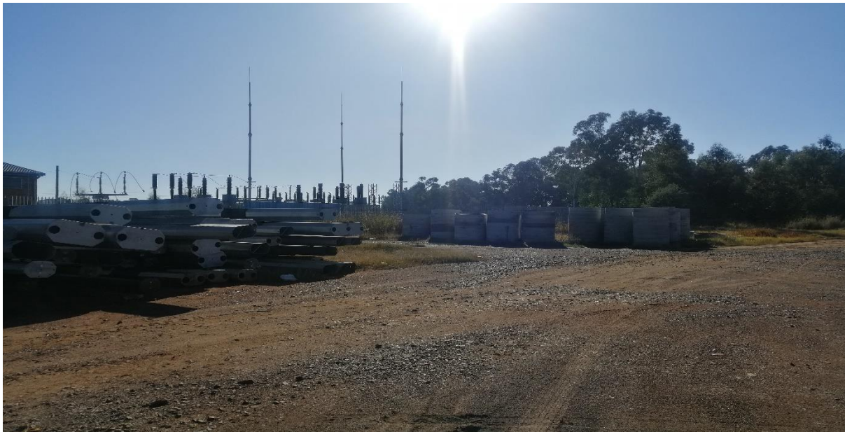
Figure 3: Material storage next to the substation.
