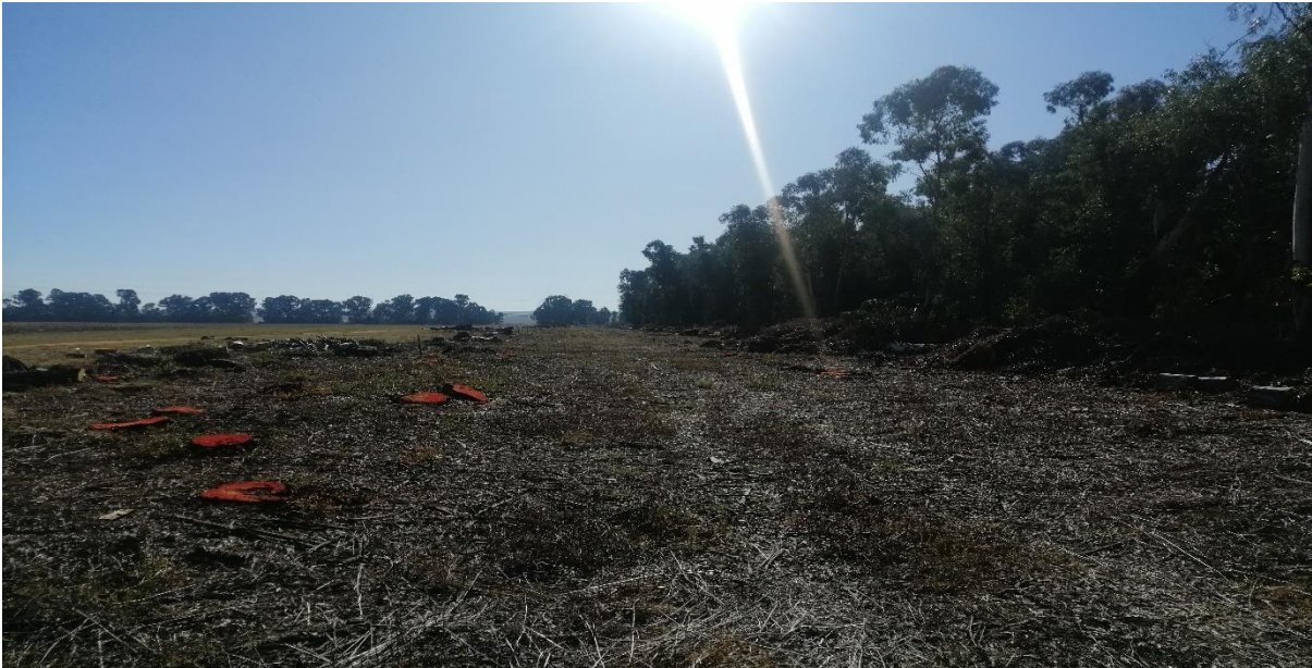
Figure 5: View of completed vegetation clearing area.
