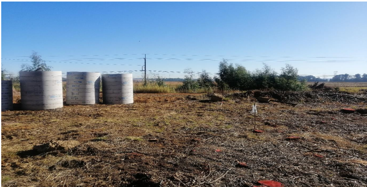
Figure 4: Material stacking in cleared construction area next to the substation.
